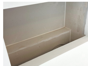
1. Hermetic sealing at top, sides and bottom. Continuous sealed base surface.
