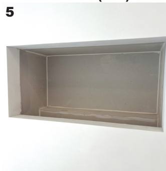
The fireplace wall must be hermetically sealed at the top, sides, and bottom.
