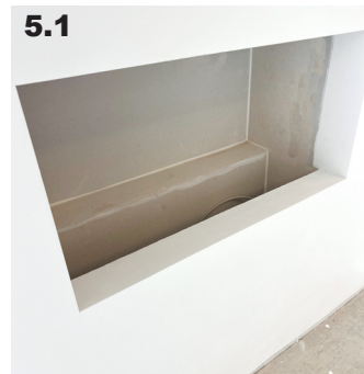
The fireplace wall must be hermetically sealed at the top, sides, and bottom.
