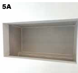
The fireplace wall must be hermetically sealed at the top, sides, and bottom.
