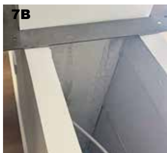
The 2 walls must be in level.
