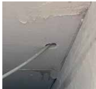
Too much space around the wiring, must be grouted.
