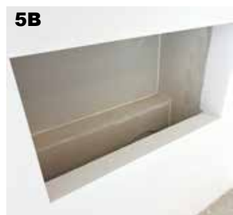
The fireplace wall must be hermetically sealed at the top, sides, and bottom.
