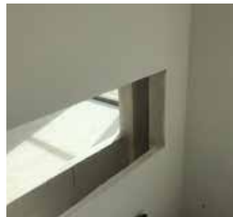
The fireplace wall is not secured against false draft in the sides.
