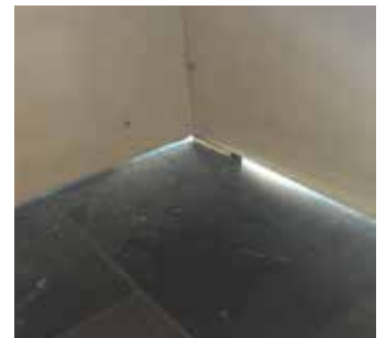
The wall is not hermetically sealed at the bottom, which can cause drafts.
